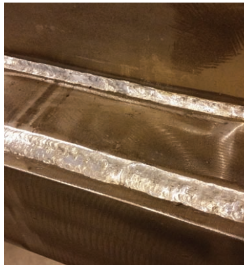
Fig. 1-4 Two different sized production fillet welds on steel made with the flux cored arc welding process. © Edward R. Bohnart
