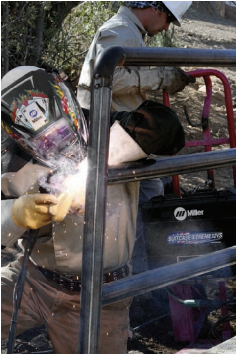
Fig. 1-6 Welding in the vertical position. © Miller Electric Mfg. Co.
